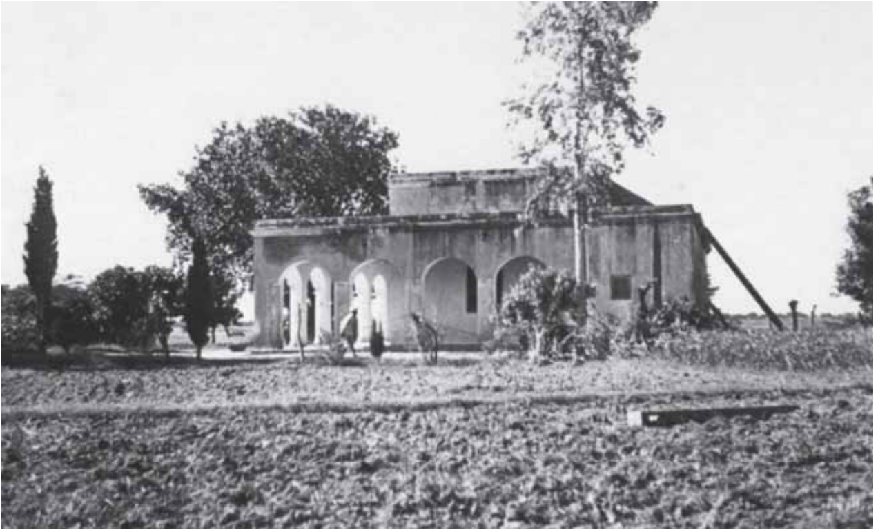
Kothi house near the Beas railway station
