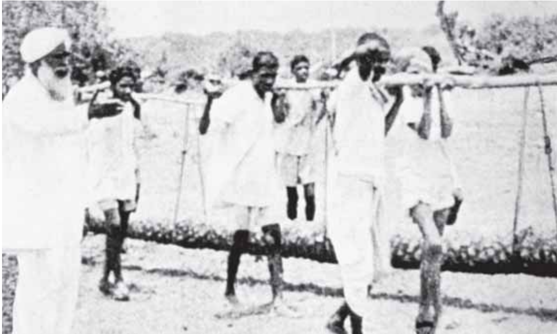
Constructing the Sawan Ashram
